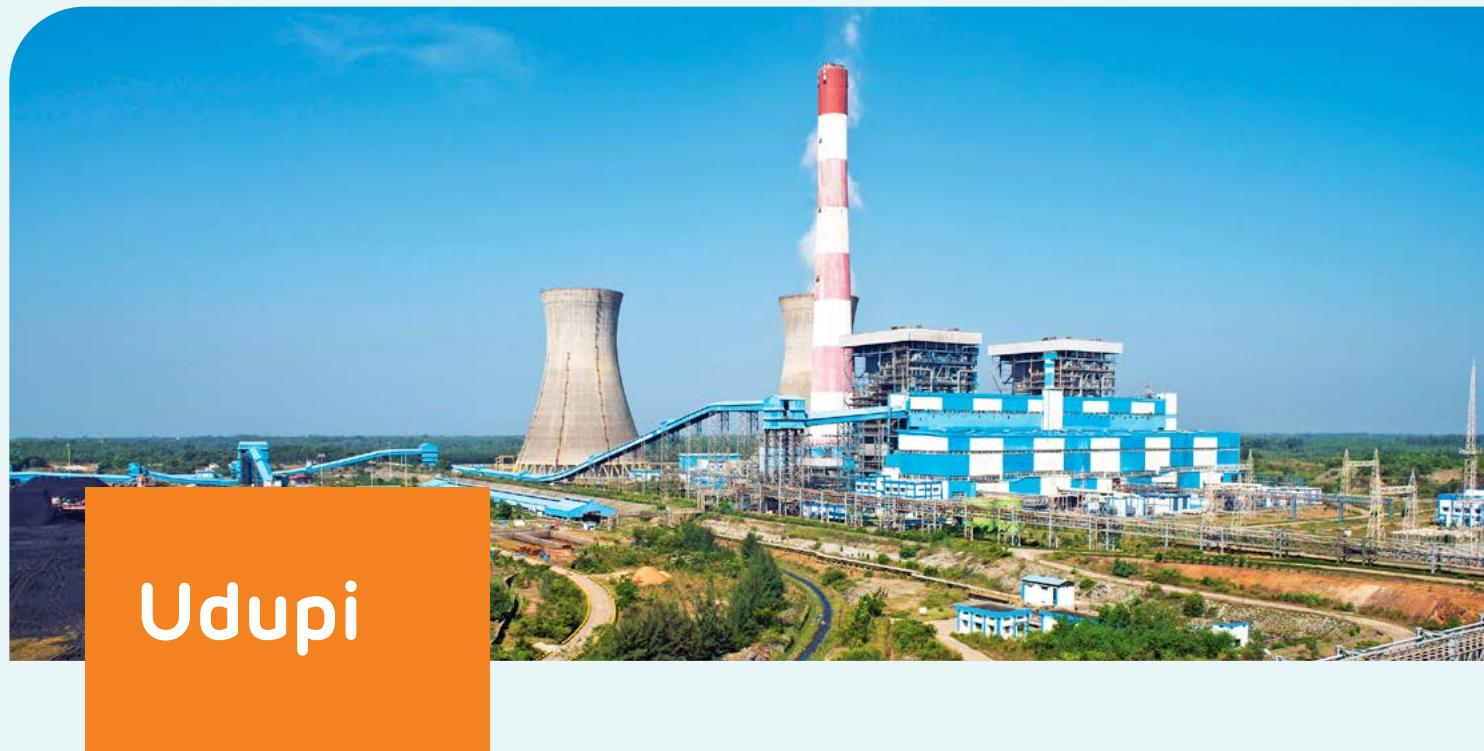
Adani Power Udupi, an imported coal-based facility, has a 1,200 MW capacity with two 600 MW subcritical units. Strategically located near key transport hubs – 15 km from the sea, 40 km from rail and air facilities – it ensures efficient coal supply, material movement, and quick access to emergency spare parts.
